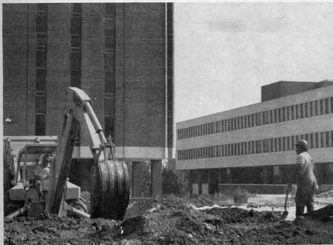
As construction nears completion, students greet the new Quadrangle between SSBE and Clark Hall with mixed reactions. An investigative report will appear in a future issue.
